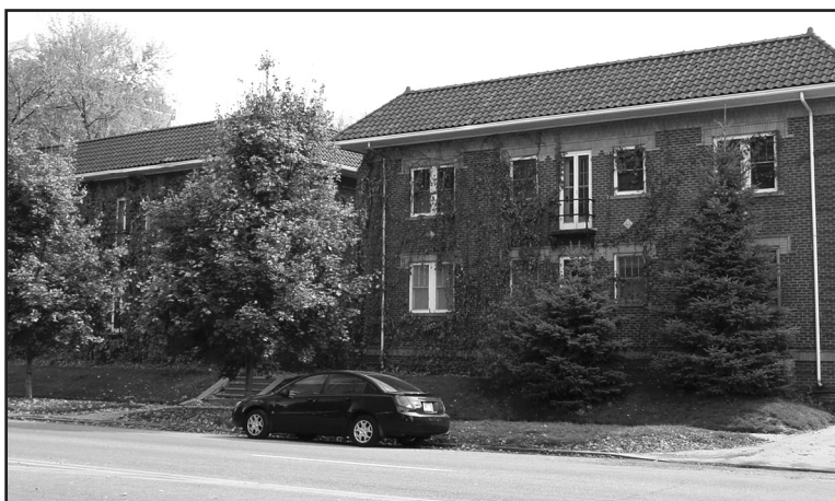
Work is under way to update the Park Court Apartments, located across from City Park in Denver.
